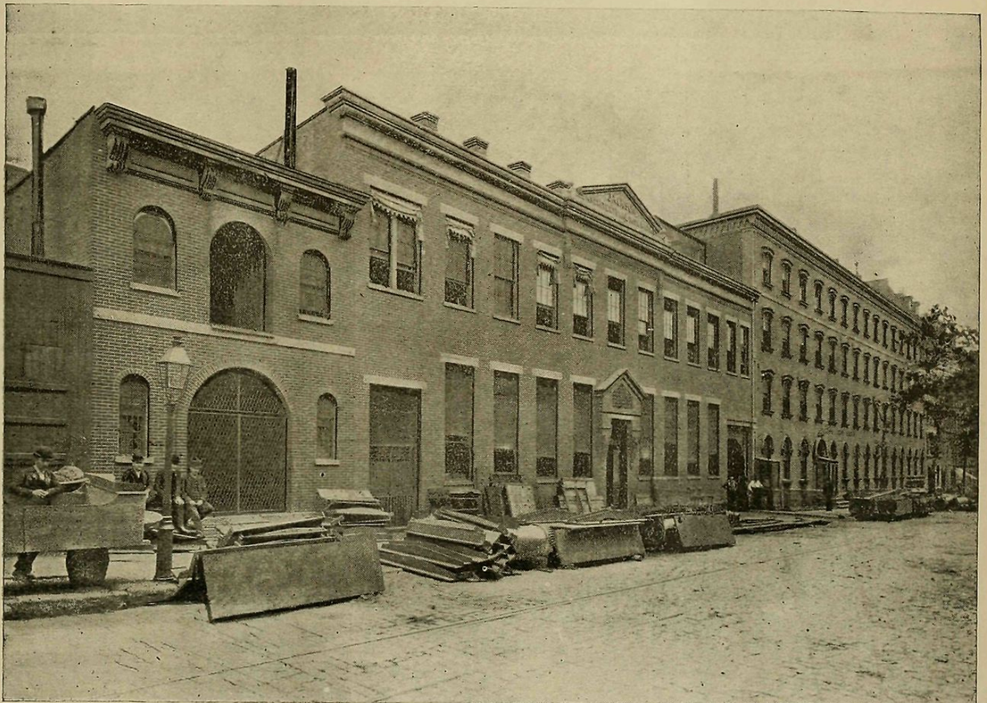
EXTERIOR OF FACTORY OF JACKSON ARCHITECTURAL IRON WORKS. 28TH STREET, EXTENDING THROUGH TO 29TH STREET.
