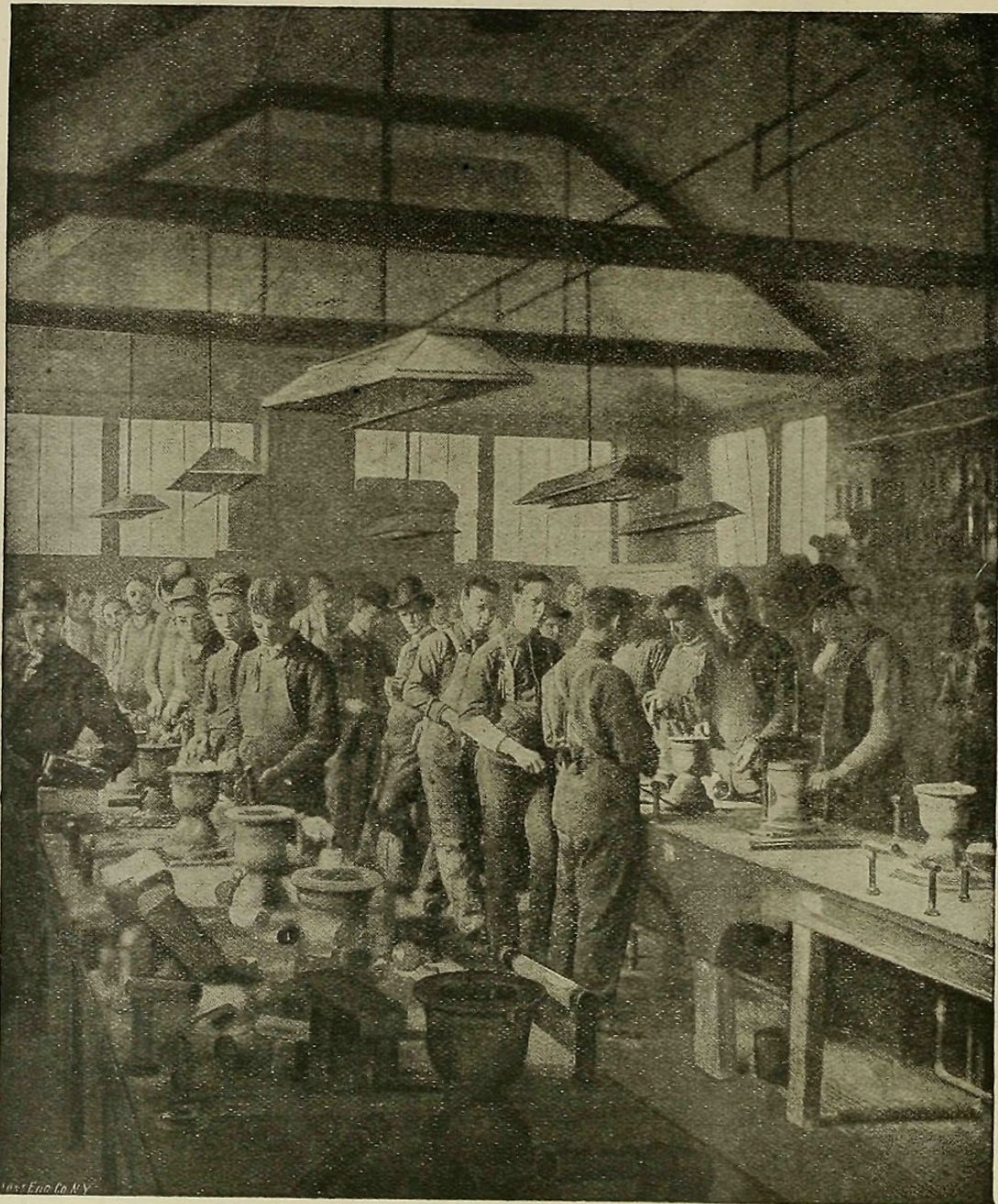
In the Plumbing Department at Col. Auchmuty's Trade Schools, visited yesterday.
