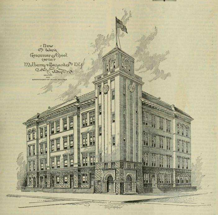
an open space in the yard at the rear and ventilated by means of exhaust flues. The first floor and all the stairways are of fire-proof construction.
