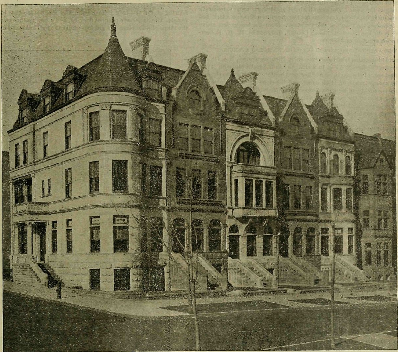
Five new houses on the northwest corner of Convent Avenue and 143d Street.
