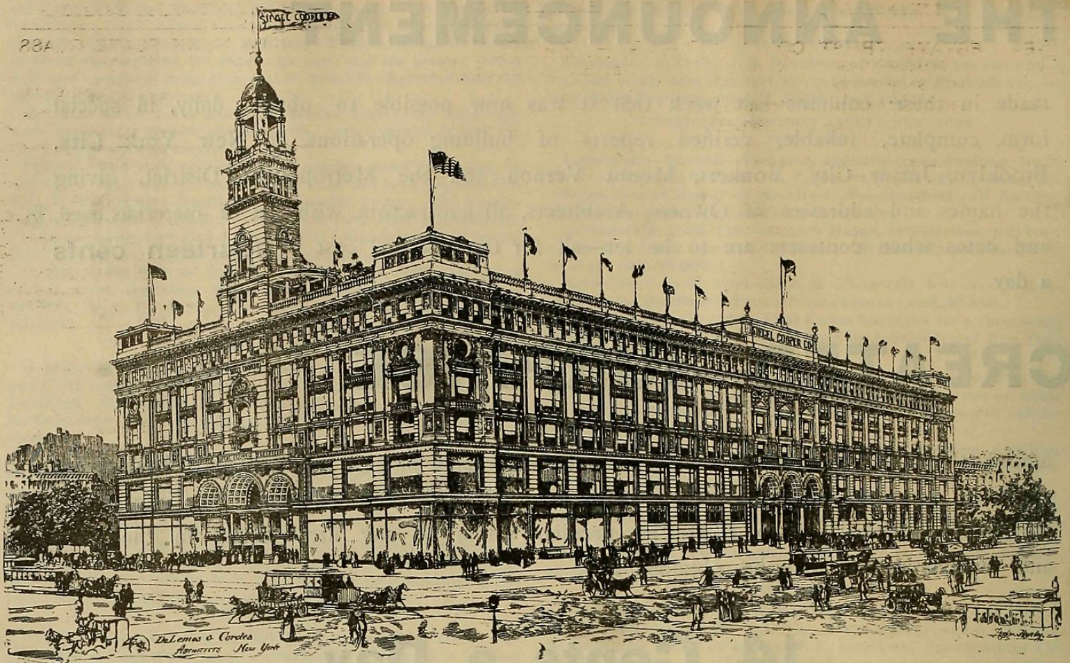
The Siegel-Cooper Building, now being erected on Sixth Avenue.
