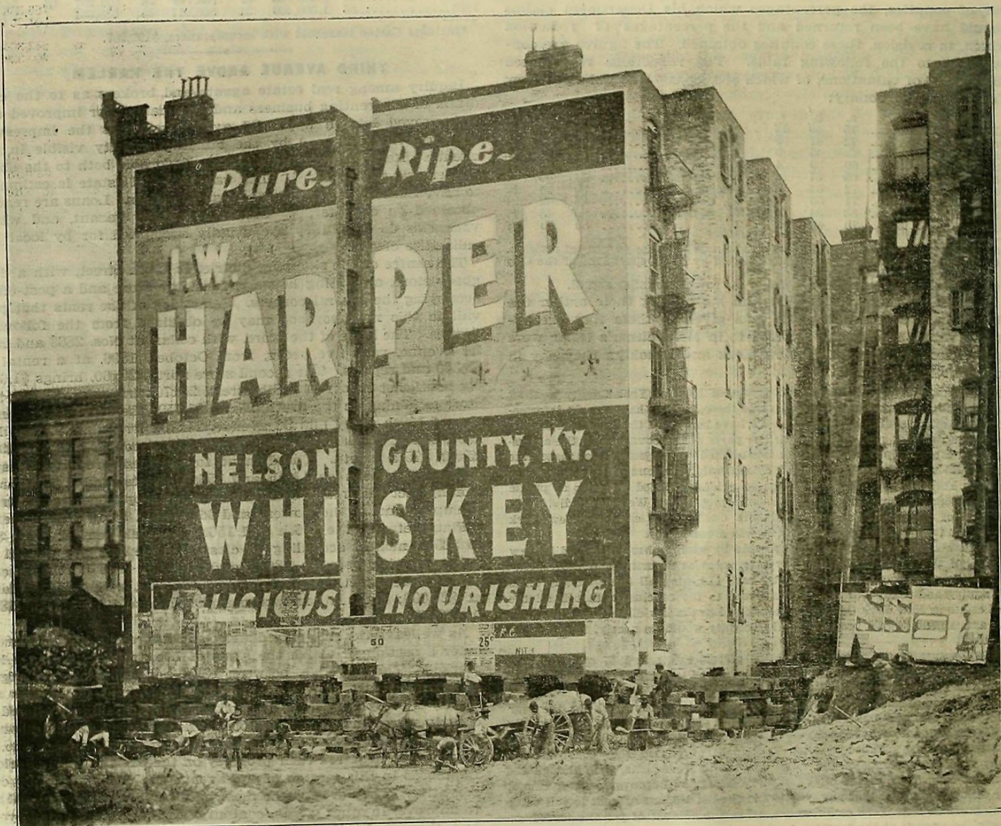
MOVING BUILDINGS AT WILLIS AVENUE AND 134TH STREET.
