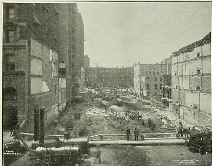
FIG. 1.—INDICATING STEAM DRILLS BORING DEEP CHANNELS CLOSE TO ADJOINING BUILDING.
