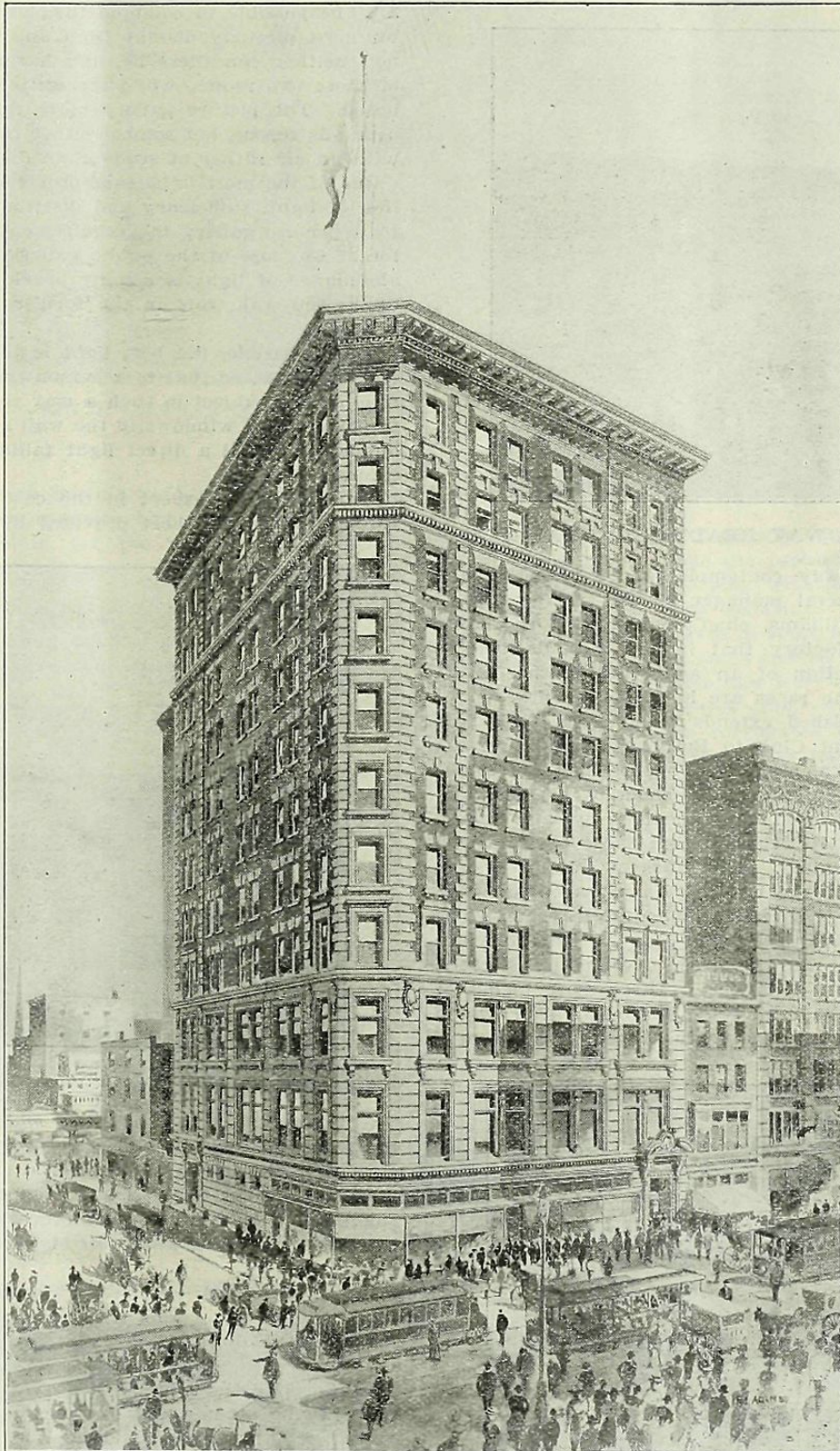
NORTHWEST CORNER 31ST ST. AND BROADWAY.
