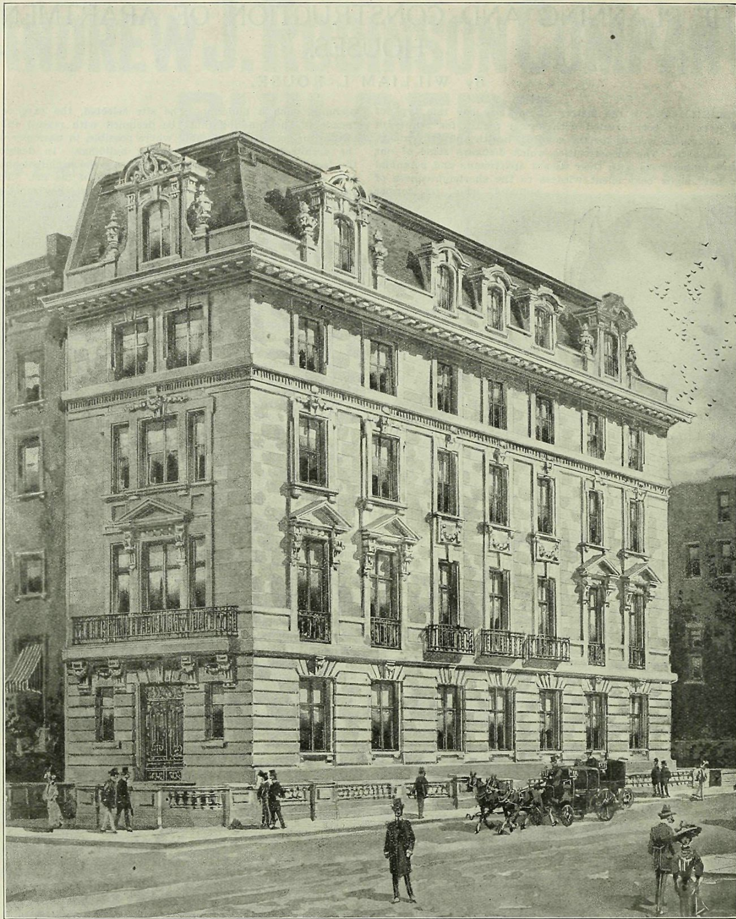
THE LATEST FIFTH AVENUE RESIDENTIAL CONSTRUCTION. House of Mr. James B. Clews, Fifth Ave. and 85th St.
