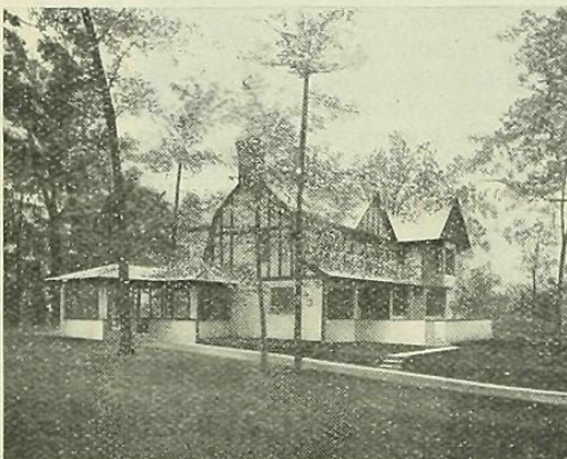
The same house completed, showing coating of Cement Stucco over walls
