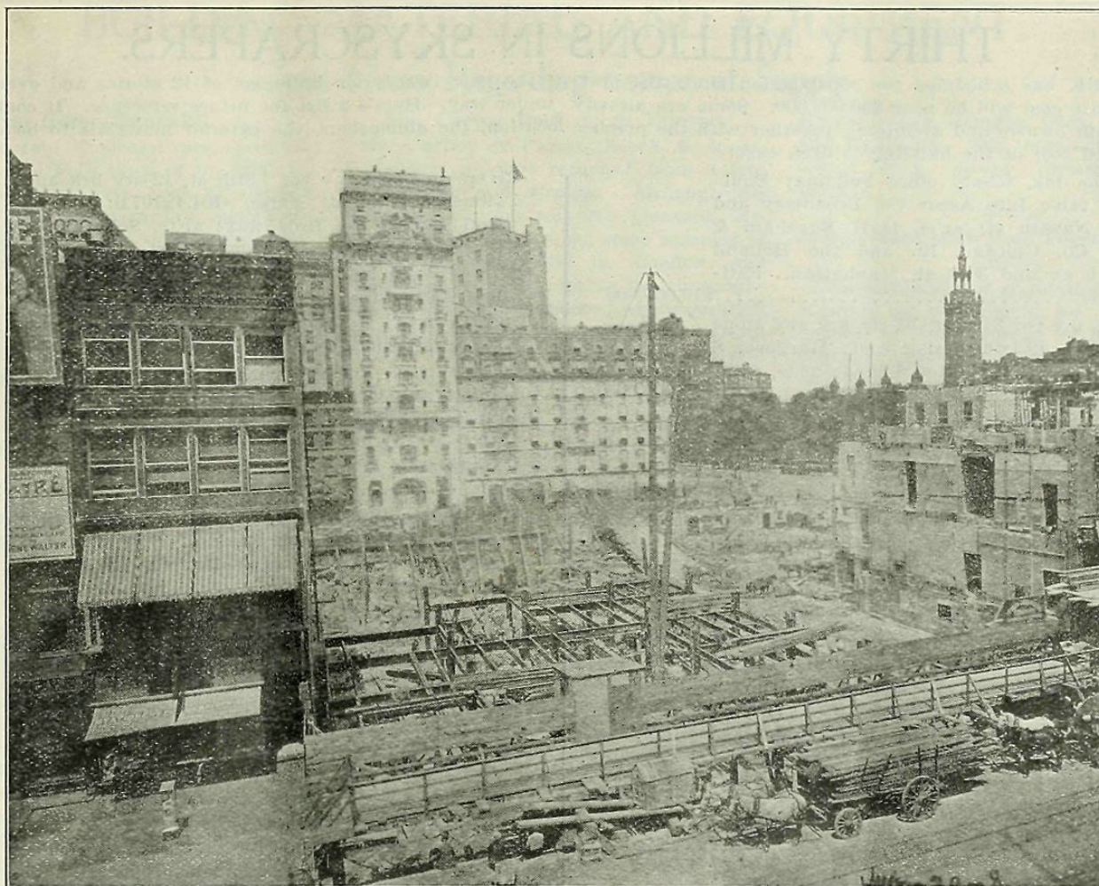
FIG. 4. VIEW OF OPERATIONS ON JULY 23.
