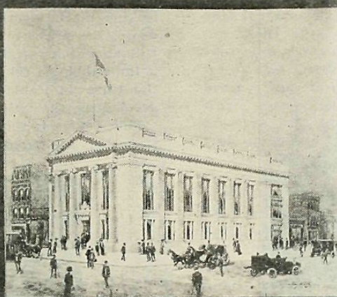
THE UNION COUNTY TRUST CO., ELIZABETH, N. J. The Hedden Construction Co., General Contractors.
