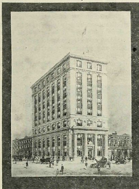
THE FIRST NATIONAL BANK, NEW BRUNSWICK, N. J. E. T. Nesbit & Co., New York, General Contractors.
