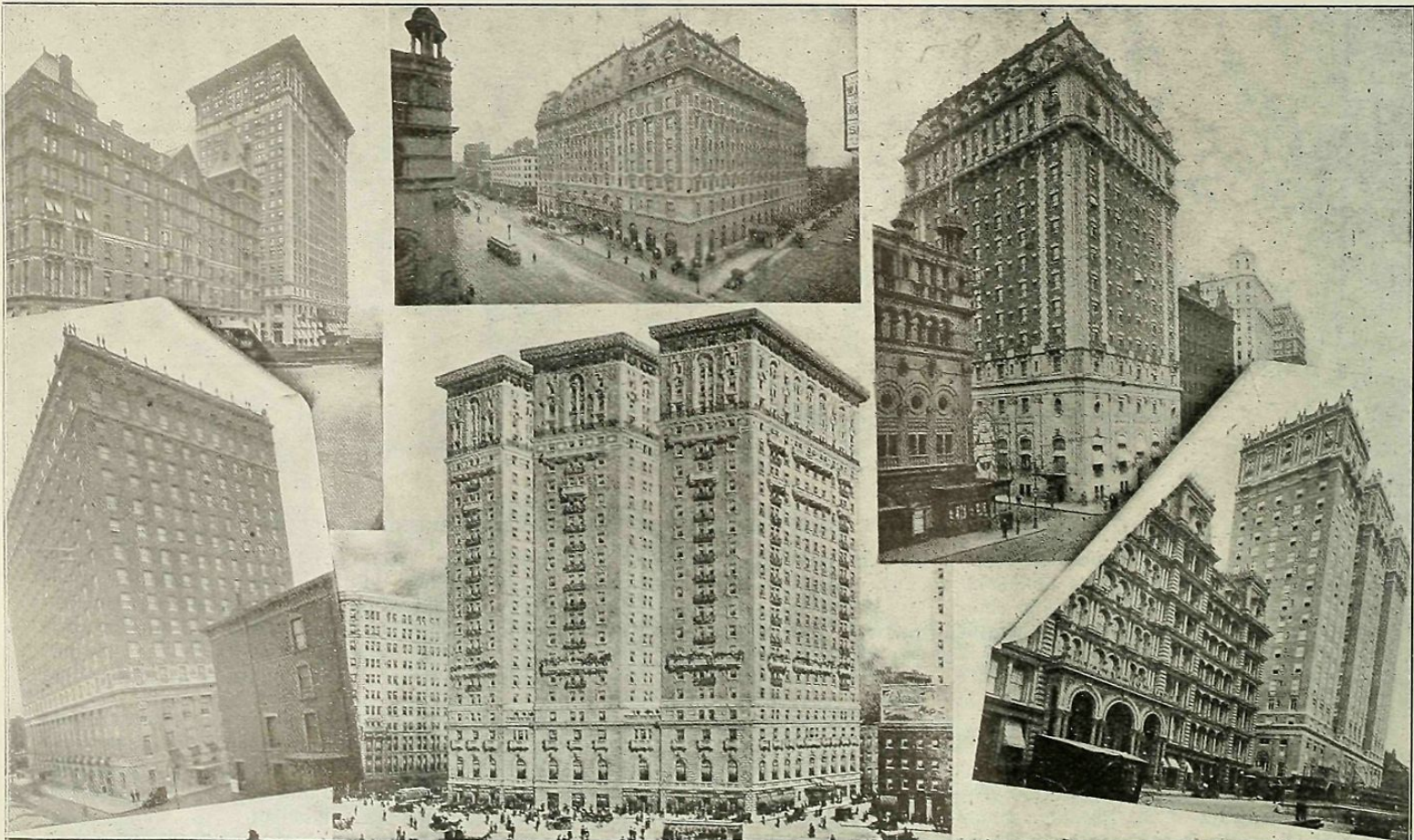
THE OLD AND THE NEW IN NEW YORK HOTEL CONSTRUCTION.
