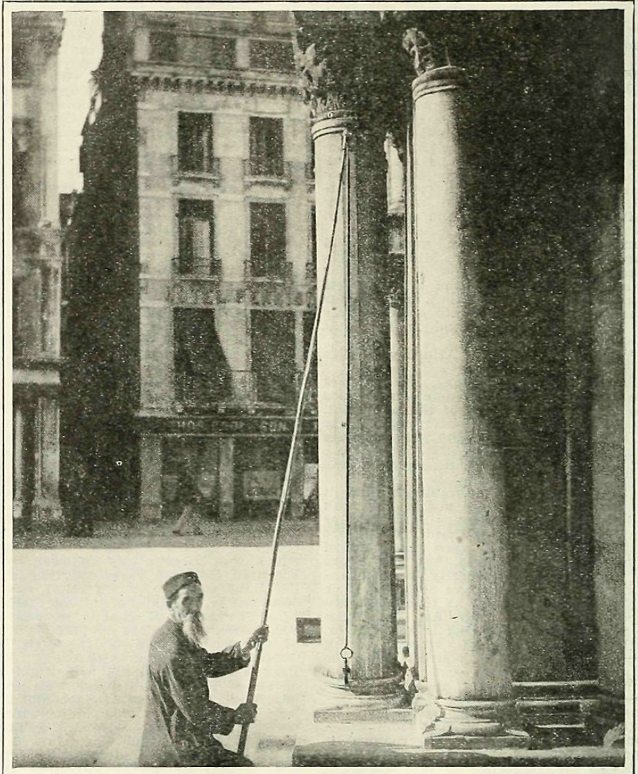
LEANING COLUMNS OF THE FACADE OF ST. MARK'S, VENICE.
