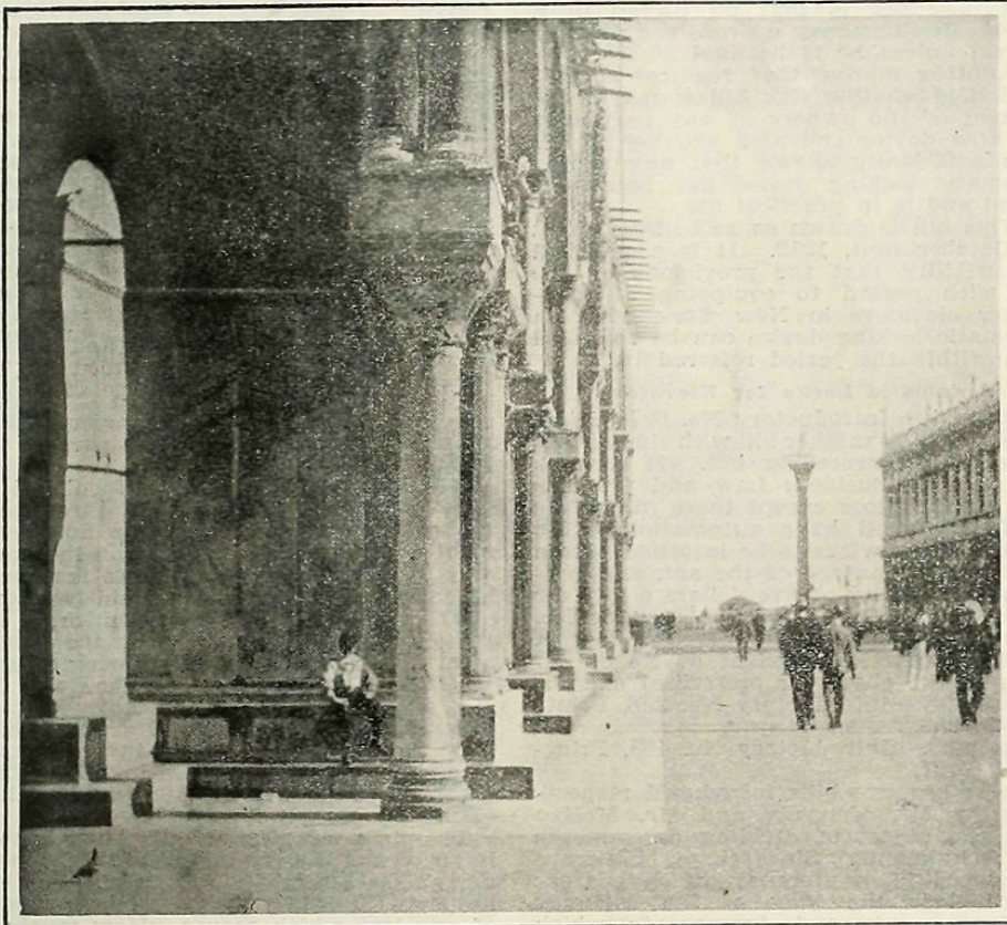
ST. MARK'S, VENICE: CURVE IN PLAN.
