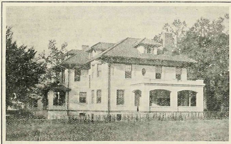
STANDARD TILE TILECRETE HOUSE PARSONS AVENUE, FLUSHING, L. I.
