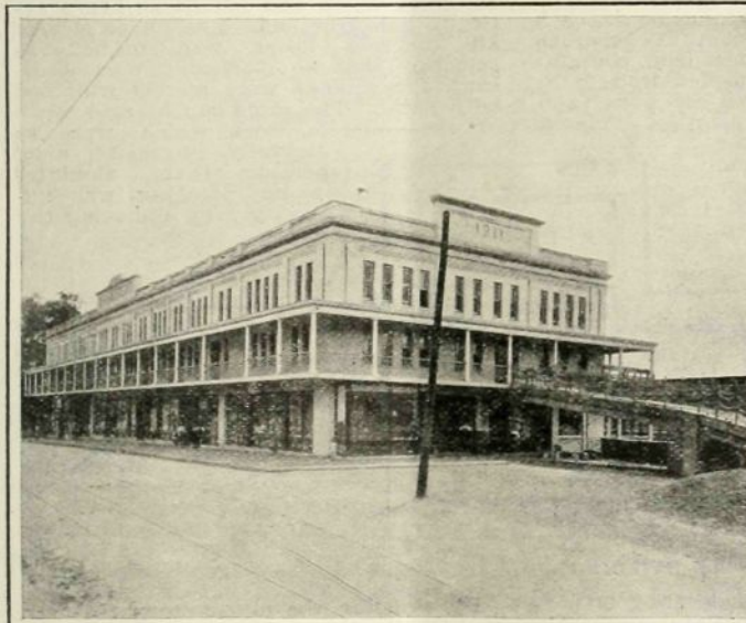
End and Side View from Street, Showing Store Front with Gallery above and Ramp from Grade to Main Floor.
