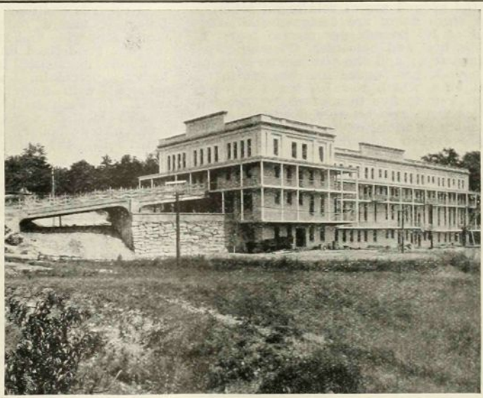
Rear Elevation, Showing the Architects' Use of Existing Grades, with Ramp to Gallery and Double Tiers of Living Porches.
