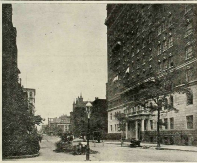
LEXINGTON AVE, LOOKING NORTH FROM GRAMERCY PARK. New Co-operative Apartment House in right foreground.
