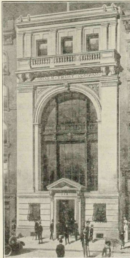
C. P. H. Gilbert, Architect. LINCOLN TRUST COMPANY BUILDING, To be erected on Madison Square.
