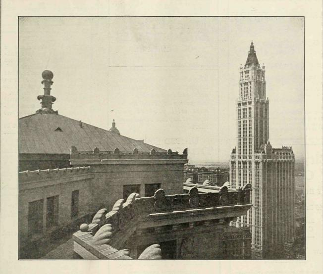
THE parapet coping and the main cornice chenaux of the Municipal Building are of Atlantic Terra Cotta, harmonizing in color and surface texture with the rough granite of the elevations.
