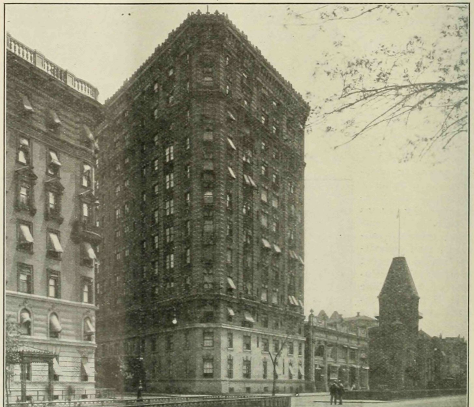
THE "SPENCER ARMS" APARTMENT HOUSE ON SHERMAN SQUARE.
