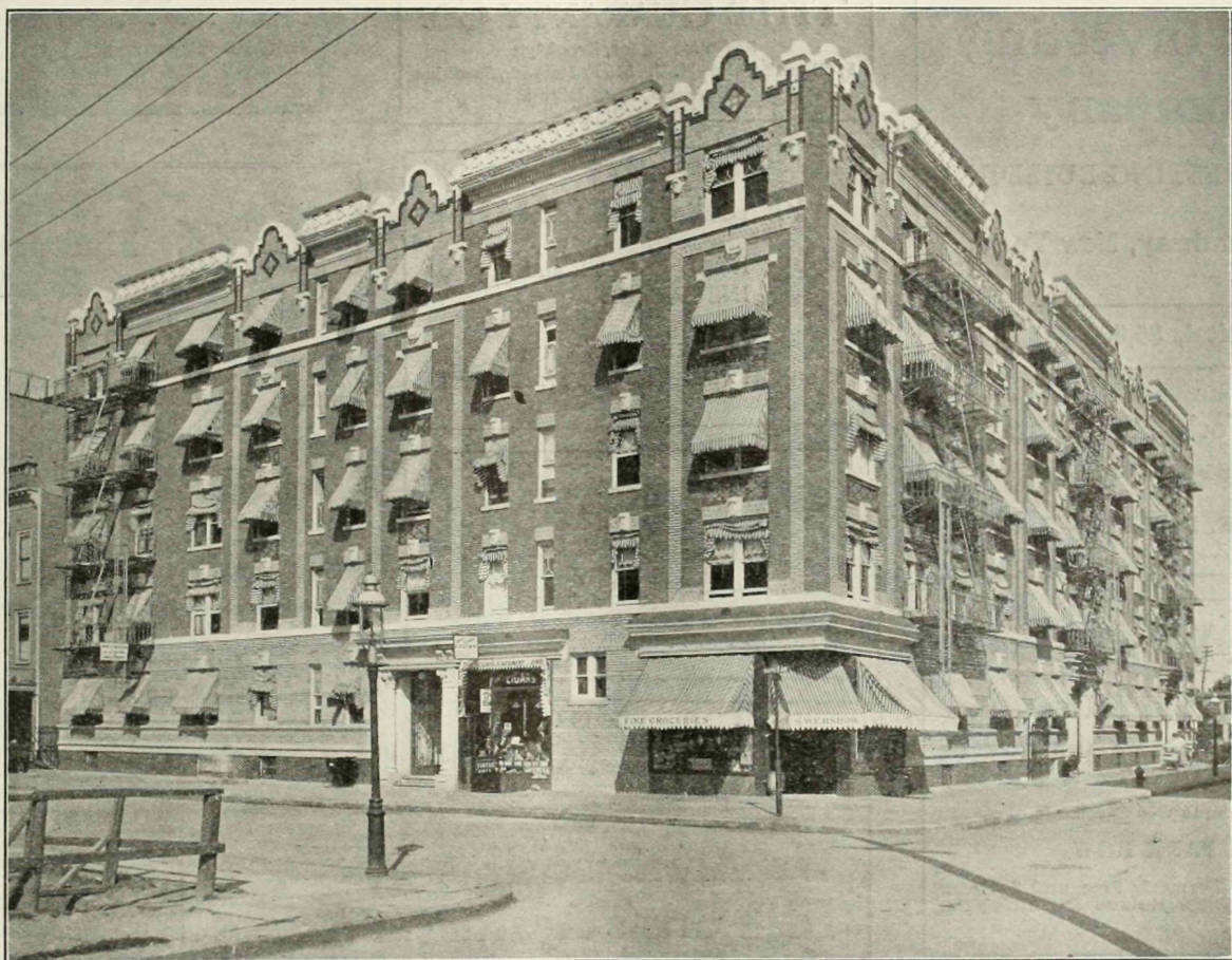
Illustration of Apartment House at 178th Street and Mapes Avenue. Henry Nordheim, Architect; James Diamond Construction Co., Builders. Building trim of Atlantic Terra Cotta in cream, enlivened with touches of green and blue.
