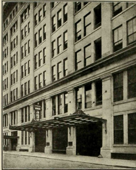
The open casements over the marquee give on the fire tower vestibules, their purpose being to prevent the accumulation of smoke in the stair enclosures.
