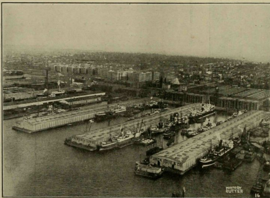
THE WATERFRONTAGE AT THE BUSH TERMINAL.
