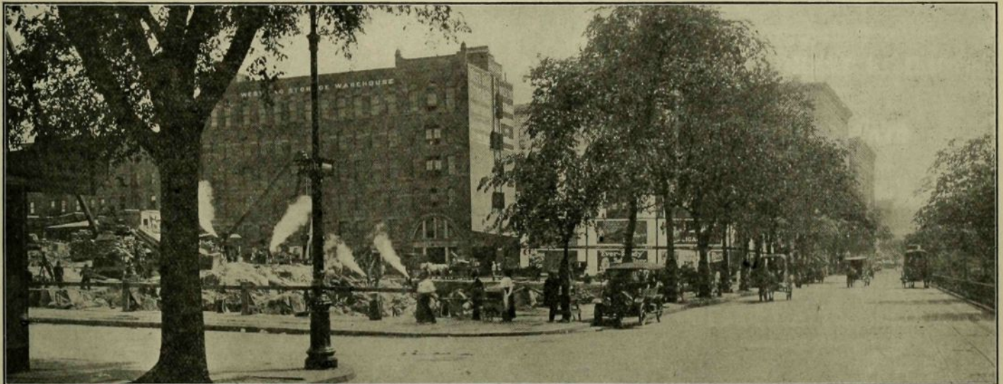
WHERE VINCENT ASTOR IS ERECTING A MILLION-DOLLAR APARTMENT HOUSE.
