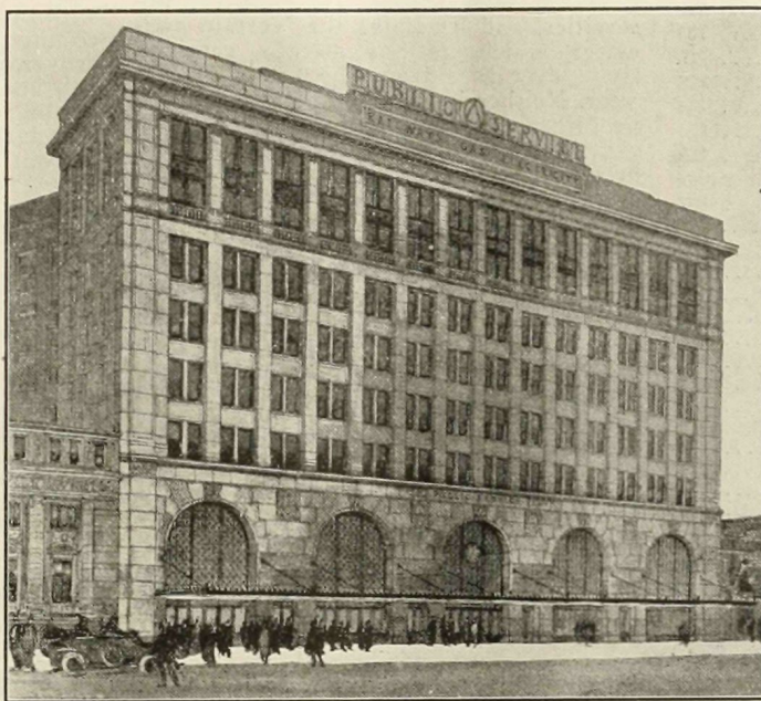
Geo. B. Post & Son, Consulting Engineers. TERMINAL BUILDING, NEWARK, N. J.
