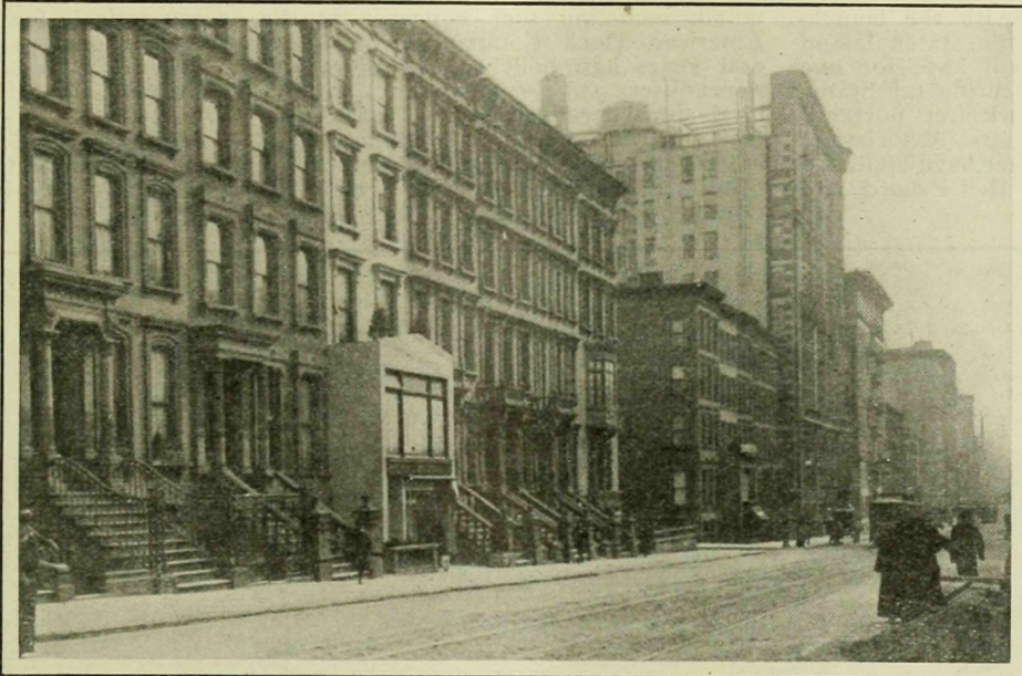
MODERNIZED DWELLING AT NO. 801 MADISON AVENUE.
