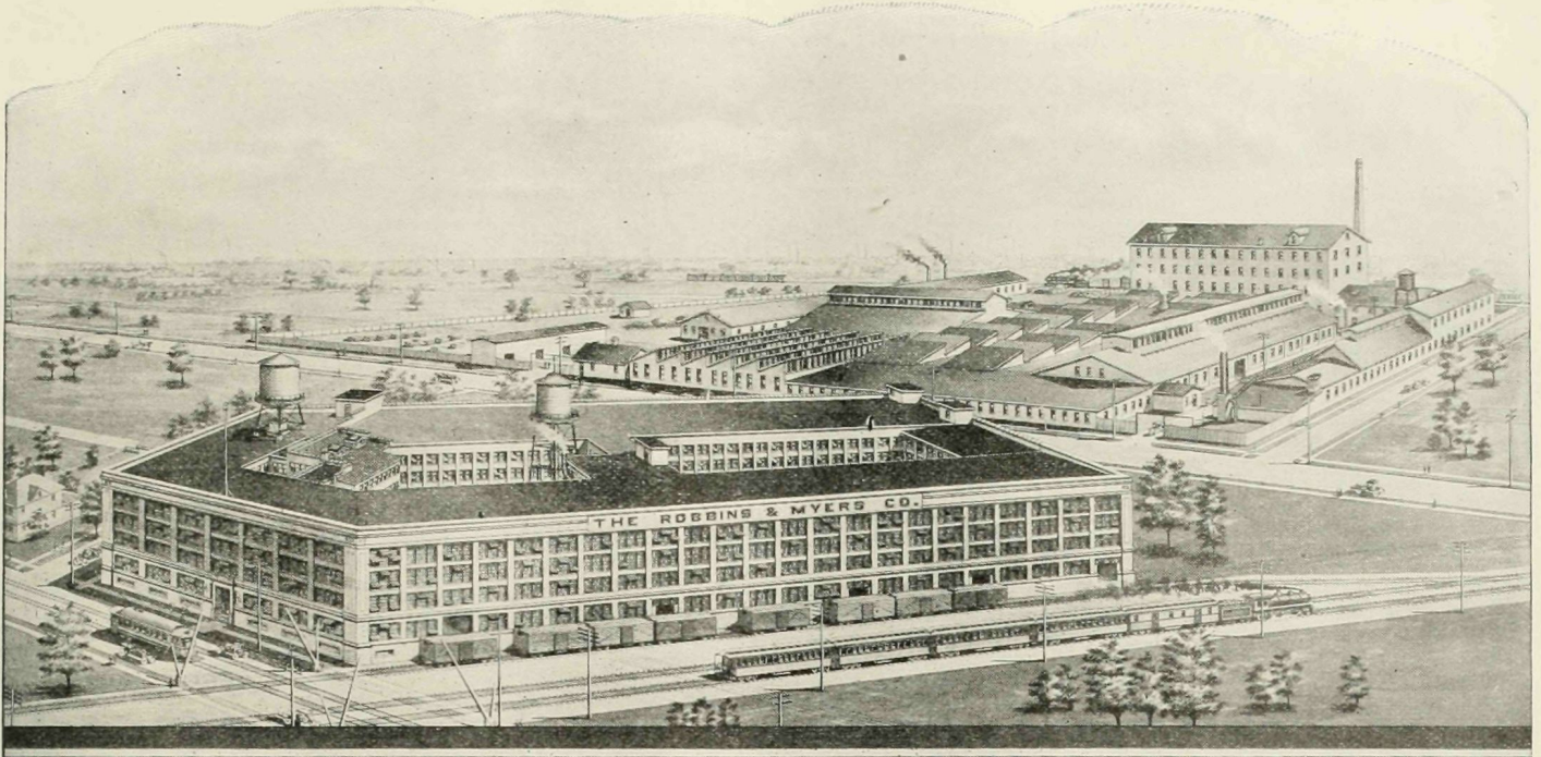
Office building and plant of Robbins & Myers Co., Springfield, Ohio. The world's largest exclusive manufacturers of small electric fans and motors. Four-story building in foreground heated with two Kewanee Smokeless Boilers each capable of heating 17,000 square feet of hot water radiation. W. E. Russ, Indianapolis, Architect; Hayes Bros. Inc., Indianapolis, Heating Contractors. Snider & Rotz, Consulting & Erecting Engineers, Indianapolis, designed the heating system.
