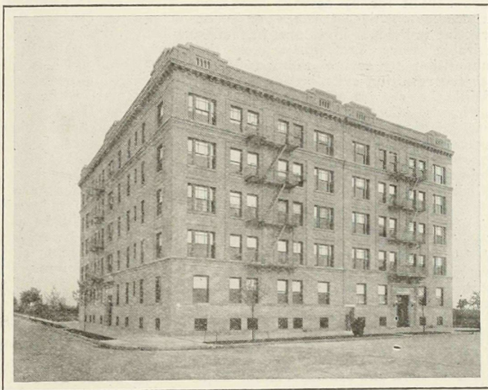
CORNER HAYES AVENUE AND 25TH STREET, ELMHURST.
