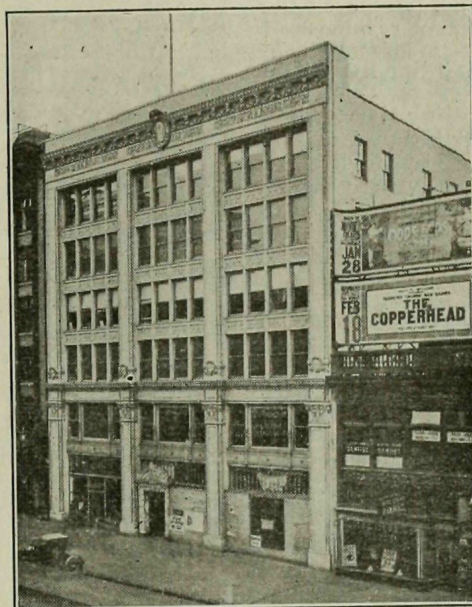
Six-Story Office Building and Store, 110-112 West 42nd Street. Owners, McCreery Realty Corp. Alfred C. Bossom, Architect. Charles T. Wills, Inc., Builder. Albin Gustafson Co., Electrical Contractors.
