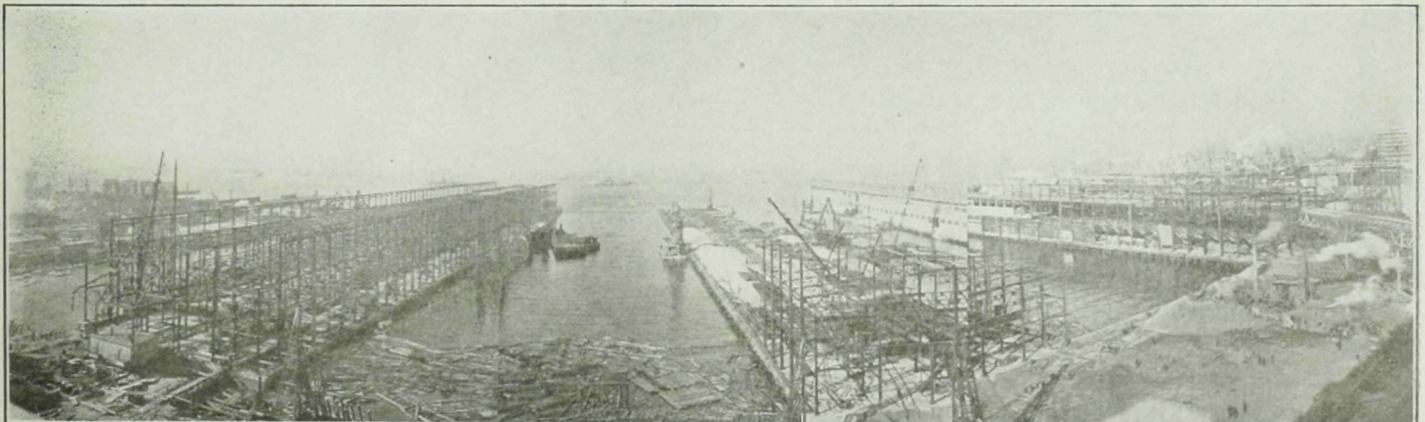
WATER FRONT CONSTRUCTION, INCLUDING BULKHEAD AND PIERS.
