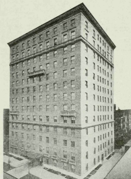
A large and modern duplex apartment at No. 246 West End Ave., New York City. Two No. 117 Kewanee Smokeless Boilers were installed.
