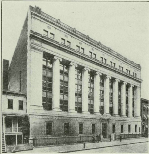
Regis High School, New York City. McGinnis & Walsh, Architects, Boston. J. Wm. Muldowney, Boston, Consulting Engineer. Kewanee Smokeless Boilers installed.
