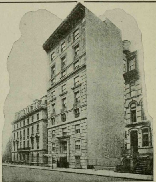
Apartment building at 3 East 85th Street, New York. Fullerton & Weaver Realty Co., Owners. Equipped with a Kewanee Smokeless Firebox Boiler and Kewanee Water Heating Garbage Burner.
